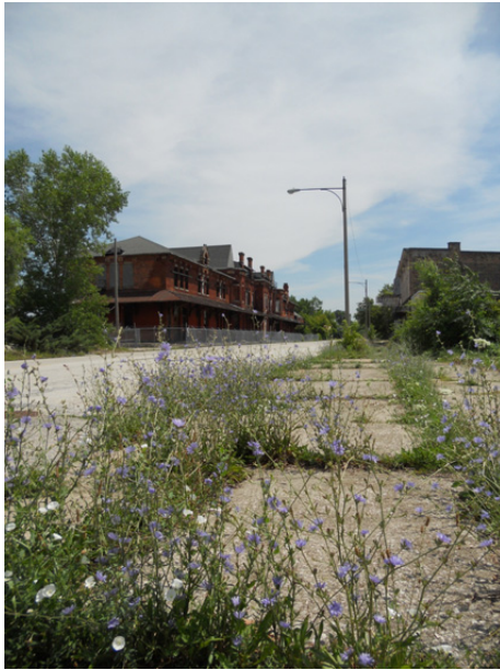
Crumbling sidewalks w/ vegetation
